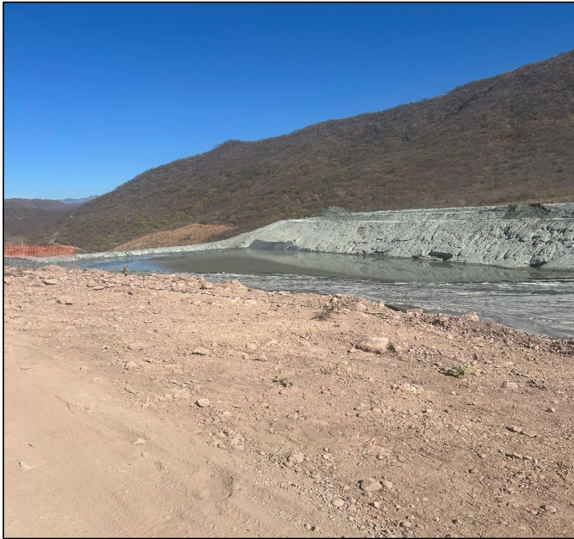
FIGURE 14.13 LINED TAILINGS STORAGE FACILITY
