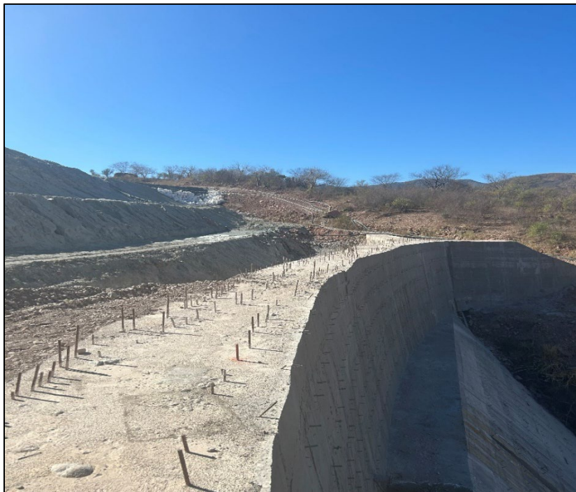
FIGURE 14.14 NEWLY CONSTRUCTED TAILINGS BERM FACILITY
